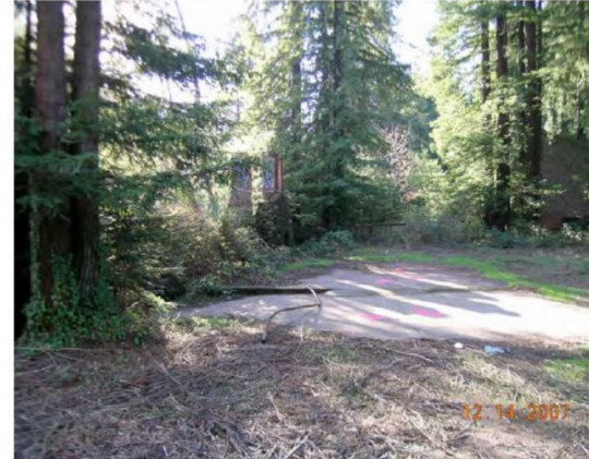
Foundations of the former resort
