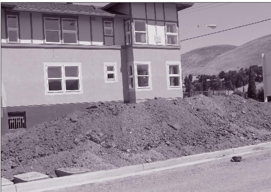
Topsoil has been removed and stockpiled before construction for later re-use in the landscape.
