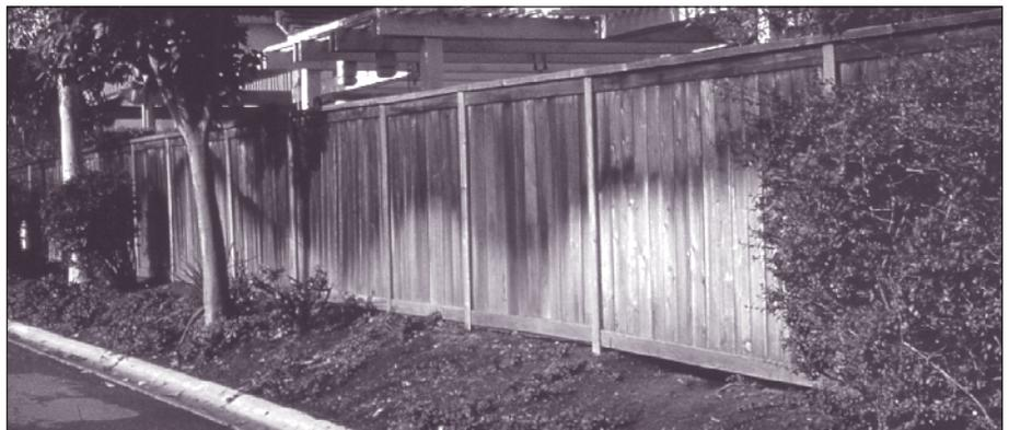
Damage to fencing from sprinkler irrigation.
