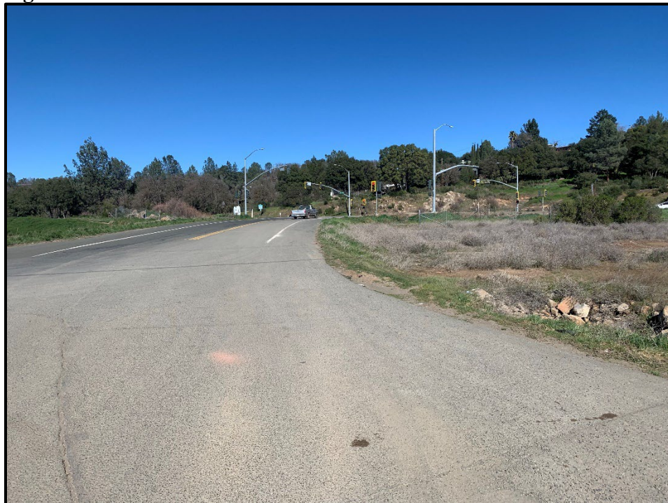
Existing SR 53/18 th Avenue Intersection
