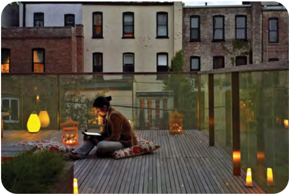
Wood Decking and Glass Guardrail
